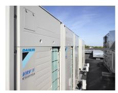
A Daikin VRV IV three-pipe heat recovery system allows zonal heating and cooling to suit different user needs.
