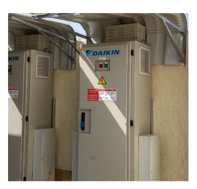
> Water Cooled Jacket for VFD Panel.. Reliable operation at high ambient conditions
