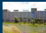
Climatisation Daikin Europe Centrale
