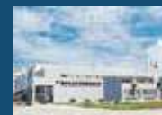
Daikin Hui Zhou Climatisation Suns
